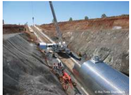
The ramp built in 2005
